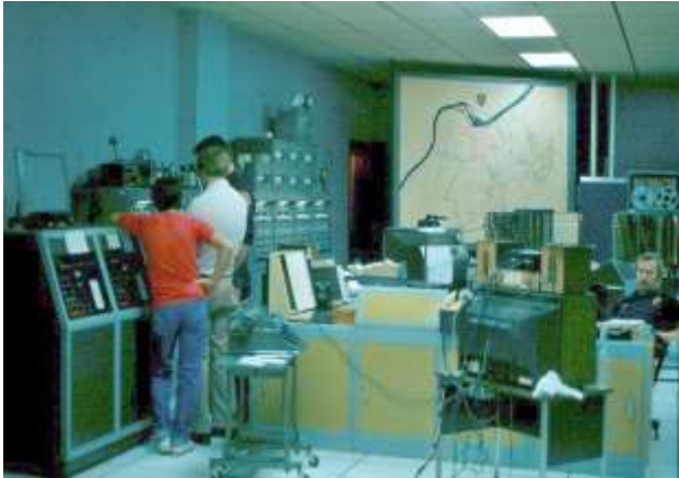
Fire Alarm Office, showing the big wall map of the city, consoles for receiving alarms from street fire alarm boxes, 2 dispatch consoles, 24 hour tape recorder, street flex-o-lines, and David Thomas watching TV.
